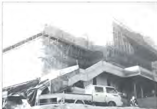
The temple has taken form, as can be seen from this photo taken December 9
